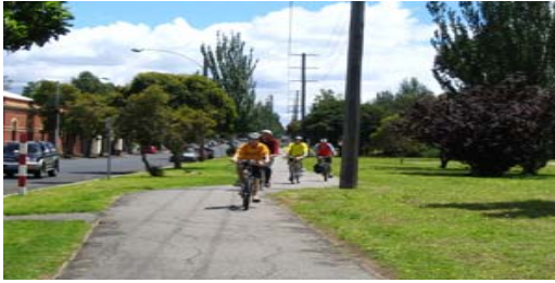
Cyclists riding on path– note deterioration at sides of path, area requires re-sheeting.
