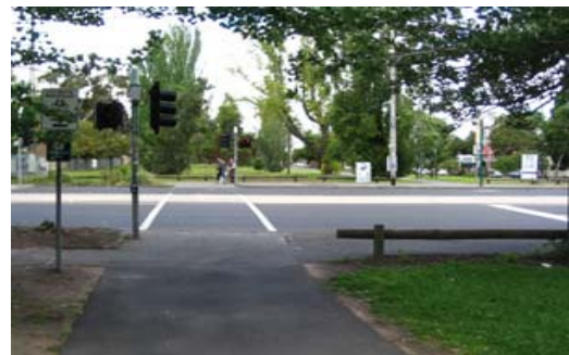
Lygon St looking east, requires extra signage denoting Shared Pathway. Caution is always required at this crossing due to Brunswick Rd intersection being just north of here...
